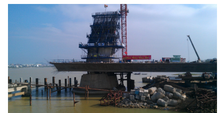
The Tran Thi Ly Bridge under construction
