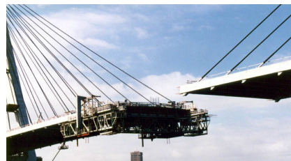
A form traveller in use during construction of a cable-stayed bridge
