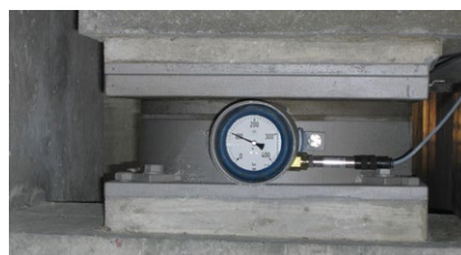
A RESTON®POT bearing with a pressure sensor, enabling bridge deck forces to be measured
