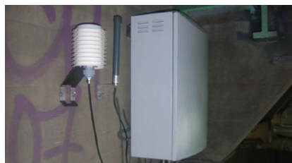
The ROBO®CONTROL Box – the heart of the monitoring system on the bridge
