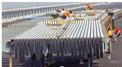
The enormous 27-gap TENSA®MODULAR joints during final assembly on the bridge due to size
