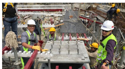
Installation of a LASTO®LRB featuring anchor plates
