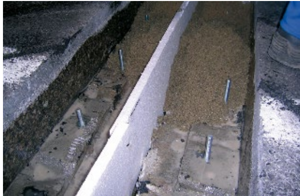
Figure 6: Forming polymer concrete base
