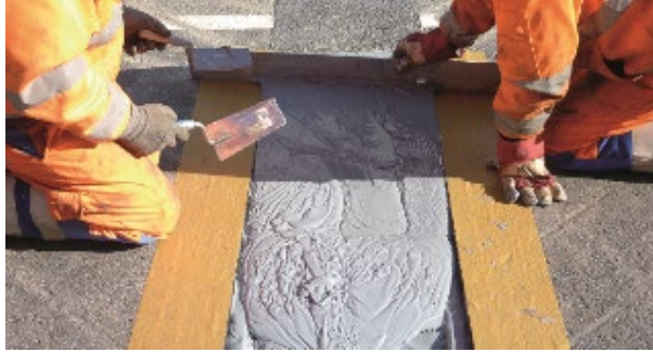
Figure 8: Precise levelling of material to road surface
