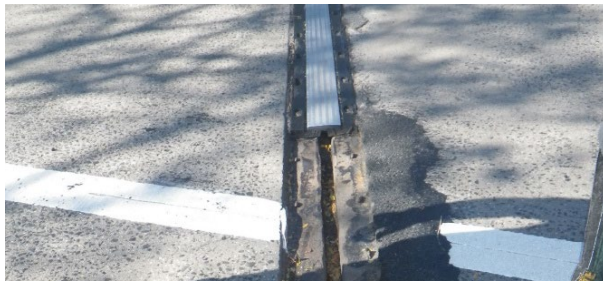
Figure 17: Existing expansion joint after removal of one particularly deteriorated section
