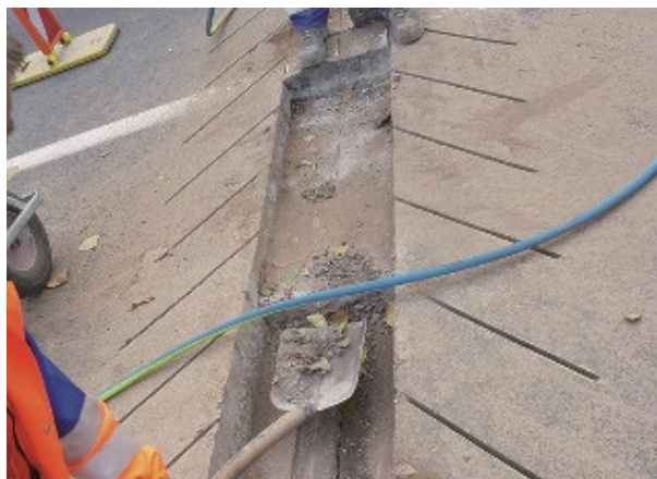
Figure 4: Removal of old joint/surfacing as needed
