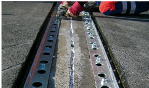
Figure 7: Fixing angles to polymer concrete base
