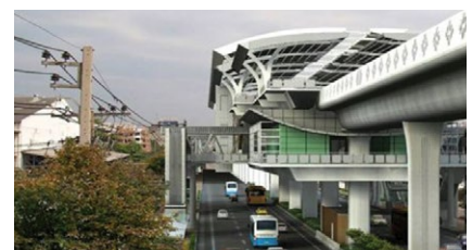
The Puchao Saming Phrai station after construction
