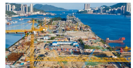
The Kai Tak Cruise Terminal during construction
