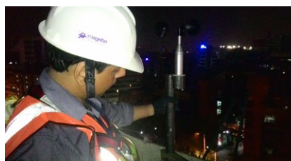
Night-installation of a wind sensor
