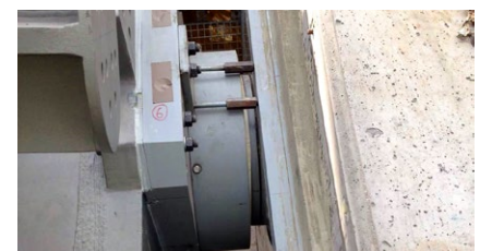
Vertically installed free sliding bearings
