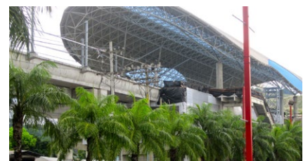
The Los Andes Metro station a couple of months before opening
