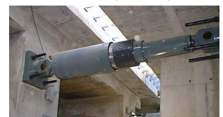
An installed RESTON®SA hydraulic damper
