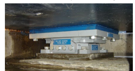
One of the 633 successfully installed bearings
