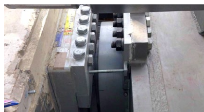
Vertically installed guided bearings
