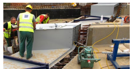
A TENSA®MODULAR joint of type LR8-RW (railway bridge joint) during installation
