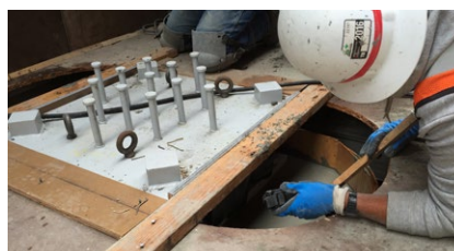
Installation of RESTON®PENDULUM Mono on terminal superstructure
