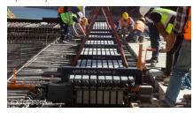
A RESTON®SPHERICAL bearing after installation
