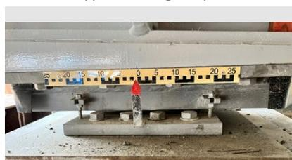
Installation of a TENSA®GRIP RS joint at one end of the new bridge
