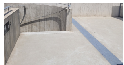
Installed POLYFLEX®SLIM PU plug expansion joint
