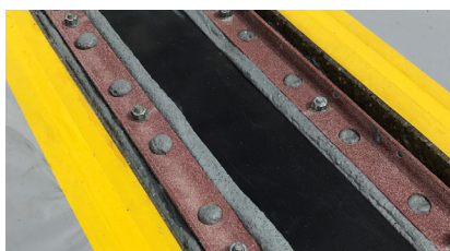
Installation of the joint with mounting inlays
