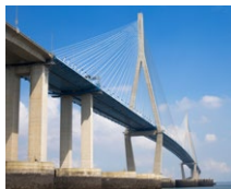
Incheon Bridge (KR)
