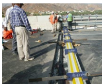
Fanja Bridge (Oman)
