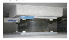
LASTO® HDRB seismic isolators are durable and low-maintenance, facilitating easy inspections.
