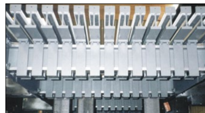
The underside of a TENSA®MODULAR joint, showing its support beams and control system
