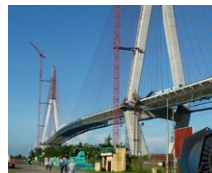
Can Tho Bridge (VN)
