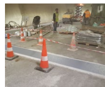
Avrasya Tunnel (TR)
