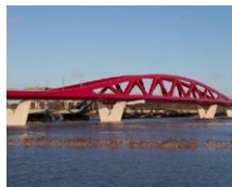
Ijssel Bridge (NL)
