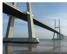
Vasco da Gama Bridge (PT)
