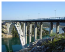
Krka Bridge (HR)
