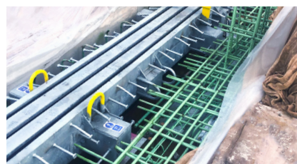
TENSA®MODULAR LR3 joint is being installed
