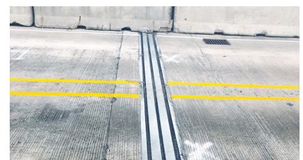
One of the installed modular joint under traffic
