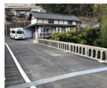
Kabutoori Bridge (JP)
