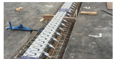
Installation of TENSA®FINGER cantilever finger joints of type RSFD-140
