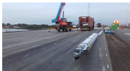
Unloading of expansion joints for the Nieuwe Hollandsebrug
