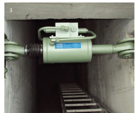
1 Performance diagram 2 Sealing system 3 Installed RESTON®STU
