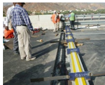
Fanja Bridge (Oman)
