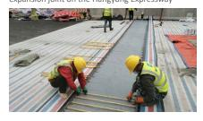
A flexible plug expansion joint after installation
