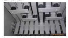
Installation of the joint featuring 11 lamellas into its recess
