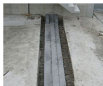
Joint prior to concreting
