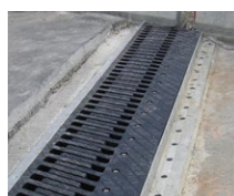
Sliding finger joint
