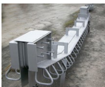
Joint ready for installation
