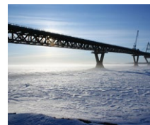
Deh Cho Bridge (CA)
