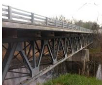
Route 9G Bridge, NY (US)
