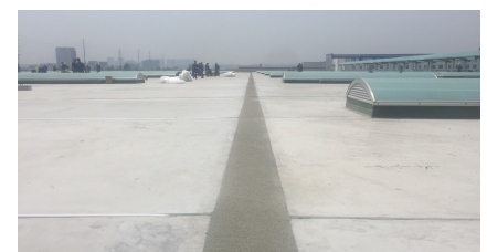
Installed TENSA®POLYFLEX®Advanced PU
