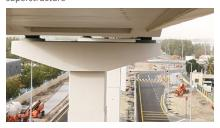
ROBO®SMART monitoring system was integrated to one of the RESTON®POT HP bearings
