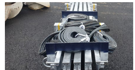
One of the modular joints before installation on site
