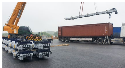
Unloading of TENSA®MODULAR LR4 joints
