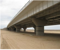
Awaza Bridge (TM)
