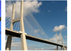
Vasco da Gama Bridge (PT)
