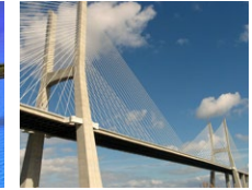
Vasco da Gama Bridge (PT)
