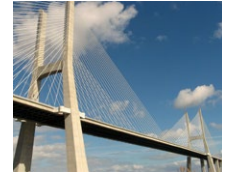
Vasco da Gama Bridge (PT)
