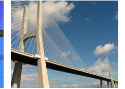
Vasco da Gama Bridge (PT)
