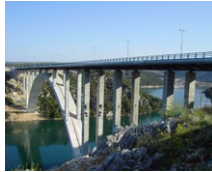
Krka Bridge (HR)
