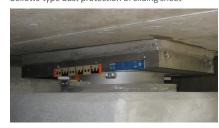
A TENSA®MODULAR expansion joint (Type LR3, with 3 movement gaps) during installation
