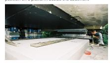
A TENSA®MODULAR joint with noise-reducing sinus plates as installed on one of the bridges
