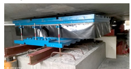
One of the installed RESTON®POT LIFT-CONTROL bearings
