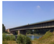
Rhine Bridge Frankenthal (DE)
