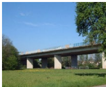
Ohrntal Bridge Öhringen (DE)
