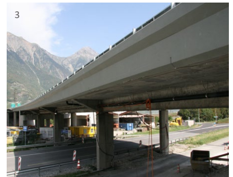
1 Testing of LASTO®HDRB bearing 2 Installed LASTO®HDRB bearing 3 Martigny bridge, Switzerland, retrofitted with LASTO®HDRB bearings
