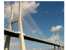
Vasco da Gama Bridge (PT)
