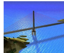
Agin Bridge (TR)
