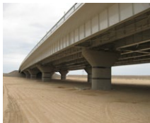
Awaza Bridge (TM)
