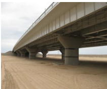
Awaza Bridge (TM)
