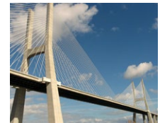
Vasco da Gama Bridge (PT)
