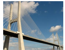
Vasco da Gama Bridge (PT)
