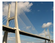
Vasco da Gama Bridge (PT)
