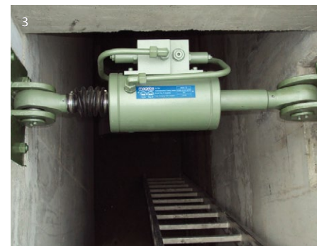
1 Performance diagram 2 Sealing system 3 Installed RESTON®STU
