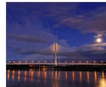
River Suir Bridge (IR)
