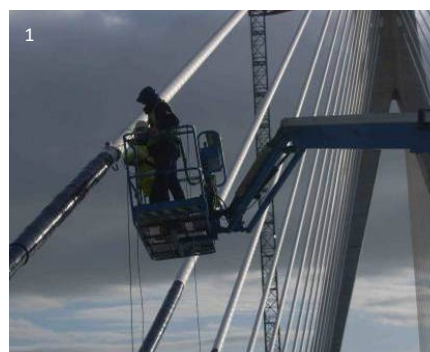
1 Installation of sensors on a cable stayed bridge
