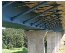
Steinbachtal Bridge (DE)
