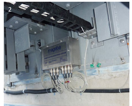
1 Installation of exceptional LR24 expansion joint 2 ROBO®CONTROL box as installed
