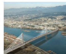
Port Mann Bridge (CA)
