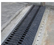
Sliding Finger Joints
