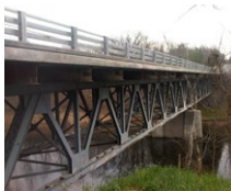
Route 9G Bridge, NY (US)
