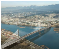
Port Mann Bridge (CA)
