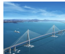
Incheon Bridge (KR)
